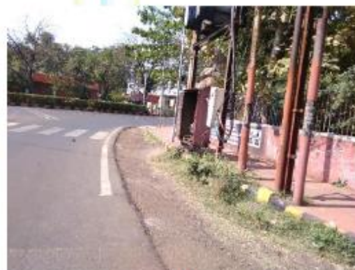
Heavy electrical utilities on the footpath causes obstruction for pedestrian movement
