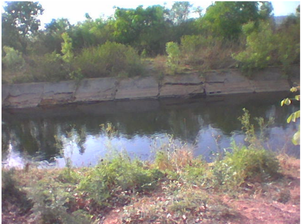
Photographs showing condition of Right Bank Canal
