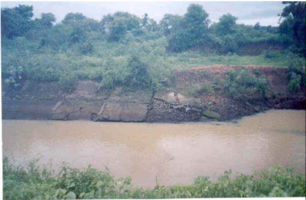
Photographs showing condition of Right Bank Canal
